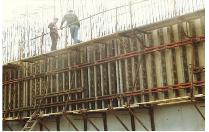
Figure 47: A view of The Marmara Ereğlisi LNG Terminal Caisson from the Construction Stage on the Ocean Going Submersible Barge of STFA (Koca Yusuf-II). Courtesy of STFA Construction Co. (from CEng. Mr. Arif Yeşiltepe - standing on the left - Private Archive)
