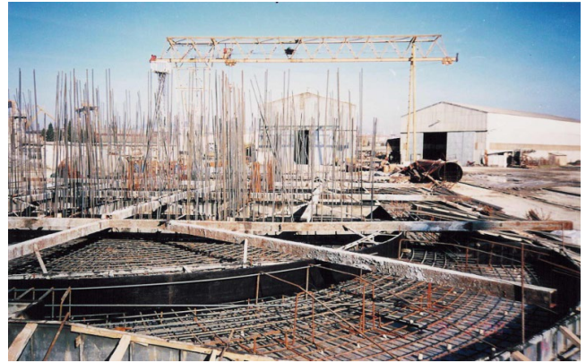
Figure 71: Figures of the Caisson Foundations
