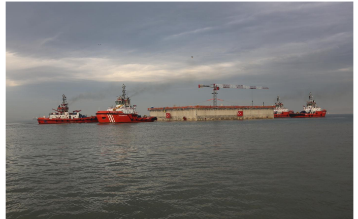
Figure 105: Initial Launching of North TF Caisson; on the right (distant two) KURTARMA-9 and KURTARMA-10 are towing the North TF Caisson, and KURTARMA-8 (right) and KURTARMA-5 (left) as Trailing Tug Boats. Courtesy of STFA Construction Co.
