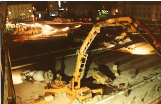
Figure 48: Concrete Casting Stage of M. Ereğlisi LNG Terminal Caisson on the Ocean Going Submersible Barge of STFA (Koca Yusuf-II). Courtesy of STFA Construction Co. (from CEng. Mr. Arif Yeşiltepe's Private Archive)
