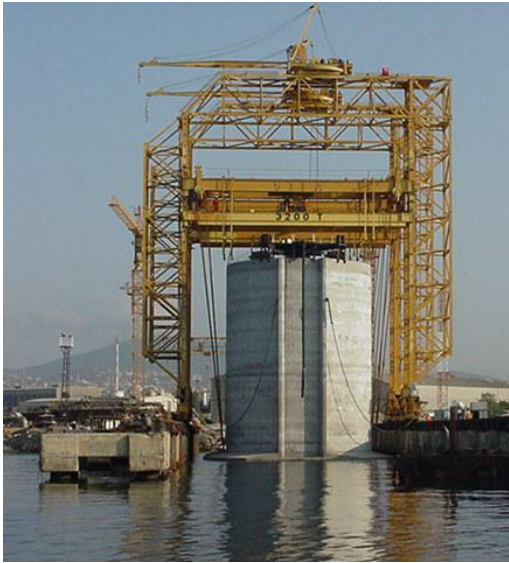
Figure 75: Handling and Lowering of the Caisson
