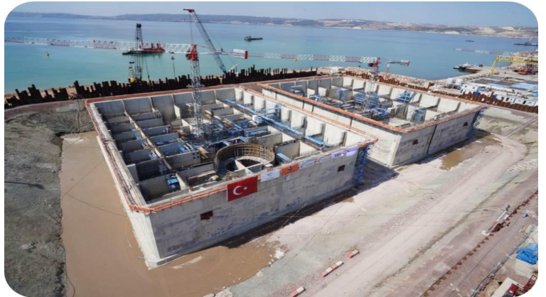
Figure 87: 3D model of the Caisson Construction at Dry Dock and water in-taking to the Dry Dock to prepare Caissons for Initial Launching. Courtesy of STFA Construction Co.
