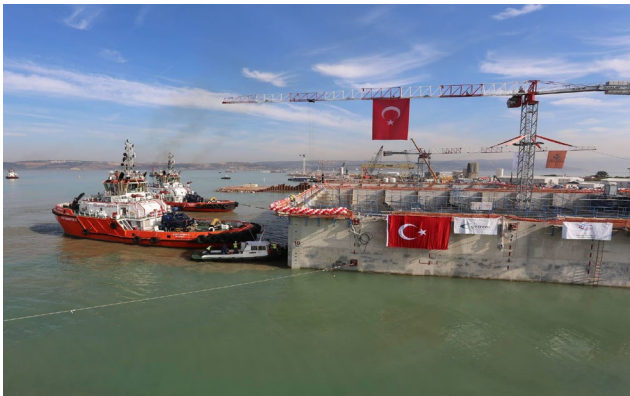
Figures 100 and 101: Hooking-up of Towing Vessels; in front Diana-II (STFA's Work Boat) in the centre and behind KURTARMA-9 and KURTARMA-10. Courtesy of STFA Construction Co.
