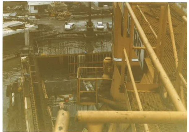
Figure 48: Concrete Casting Stage of M. Ereğlisi LNG Terminal Caisson on the Ocean Going Submersible Barge of STFA (Koca Yusuf-II). Courtesy of STFA Construction Co. (from CEng. Mr. Arif Yeşiltepe's Private Archive)
