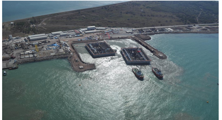
Figures 100 and 101: Hooking-up of Towing Vessels; in front Diana-II (STFA's Work Boat) in the centre and behind KURTARMA-9 and KURTARMA-10. Courtesy of STFA Construction Co.
