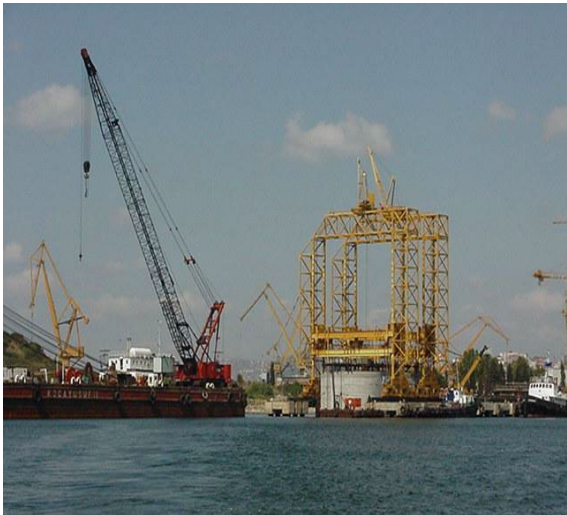
← ↑ Figure 76: Lowering, Handling and Floating of the Caissons
