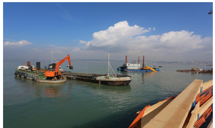
Figure 142: Dredging by Back-Hoe Deep Dredger. Courtesy of STFA Construction Co.
