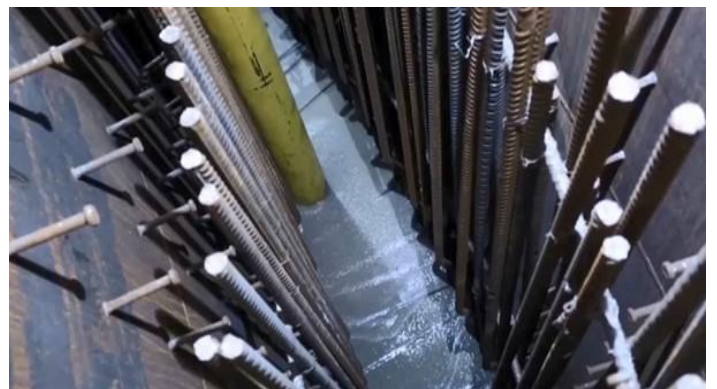
Figure 148: Casting of SCC with Tremie Pipes
