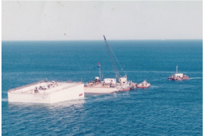
Figure 52: Submerging operation is ongoing for STFA's Submersible Barge (Koca Yusuf II), therefore the Water Intake Caisson is moving towards its planned location at Marmara Ereğlisi LNG Terminal. Courtesy of STFA Construction Co. (from CEng. Mr. Erkan Çırak's Private Archive)
