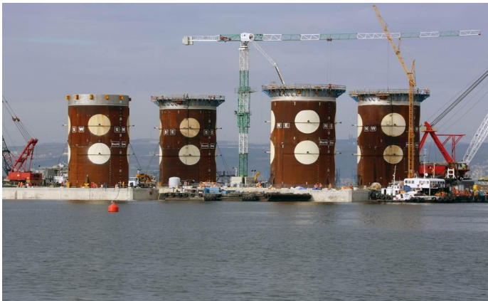
Figure 132: The Caissons are ready to Hook-Up and Tow at Wet Dock.
