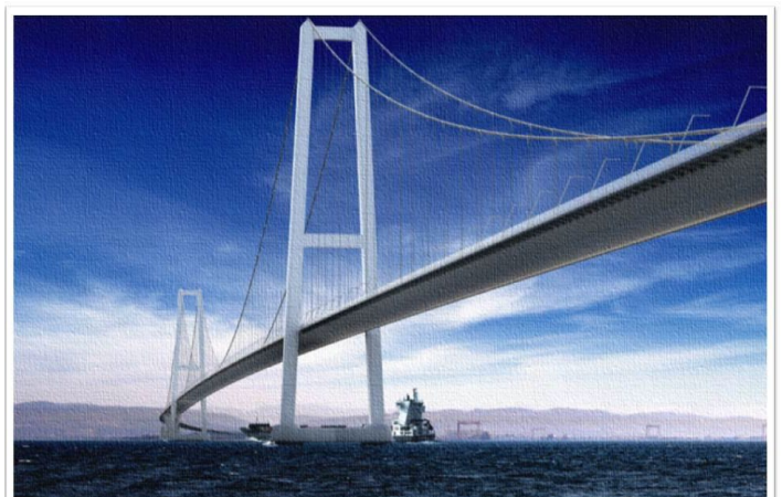
Figure 83: Animated Figure from the Design Stage of the Osmangazi Suspension Bridge. Courtesy of Concessionaire OTOYOL YATIRIM ve İŞLETME INC.
