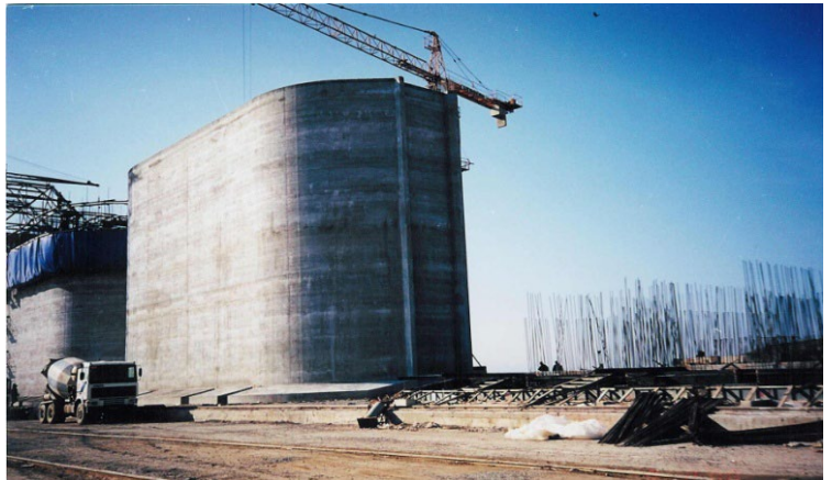
Figure 58: A photograph from the Caisson Construction stage
