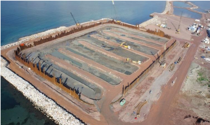
Figure 140: Dewatering and Excavation of Dry Dock. Courtesy of STFA Construction Co.
