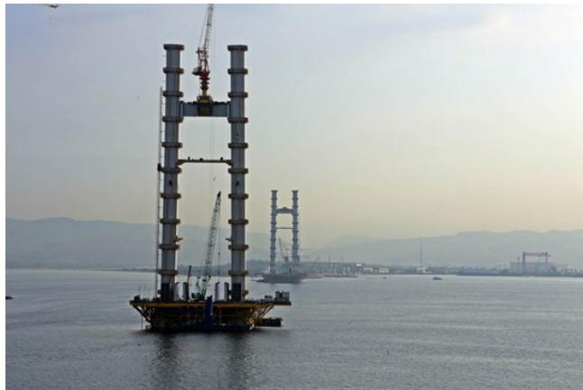
Figure 29: Caissons in Marine Engineering
