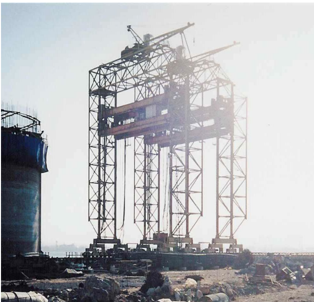
Figure 65: DEVE Heavy Crane from the Caisson Construction Yard, and Lifting Rope Configuration for the Caisson
