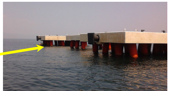
Figure 88: Towing of Caissons from Dry Dock (Hersek/Altinova/Yalova) to Wet Dock (Kaytazdere/Yalova); Initial Launching. Courtesy of STFA Construction Co.
