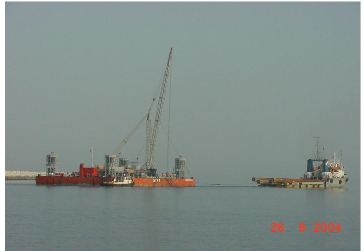
Figure 10: Towage of Hollow-Shaped Hergeleci Jack-up Barge. Courtesy STFA Construction Co.
