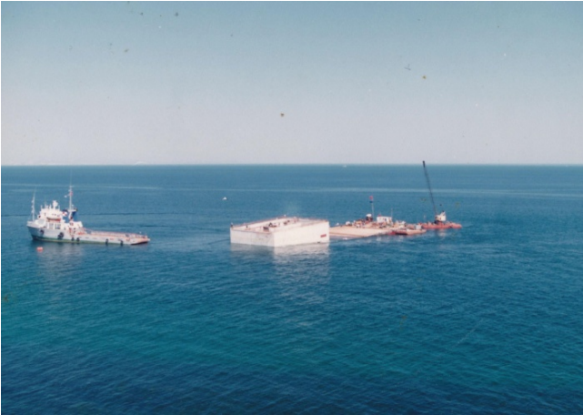
Figure 52: Submerging operation is ongoing for STFA's Submersible Barge (Koca Yusuf II), therefore the Water Intake Caisson is moving towards its planned location at Marmara Ereğlisi LNG Terminal. Courtesy of STFA Construction Co. (from CEng. Mr. Erkan Çırak's Private Archive)
