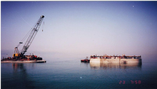
Figure 77: Floating, Towing and Placement of the Caisson
