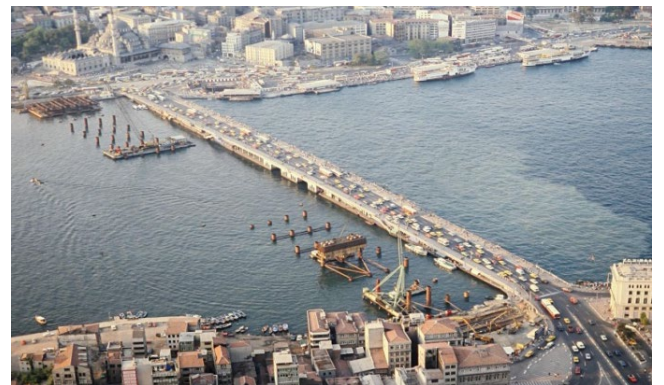
Figure 34: Galata Bridge in Construction Stage
