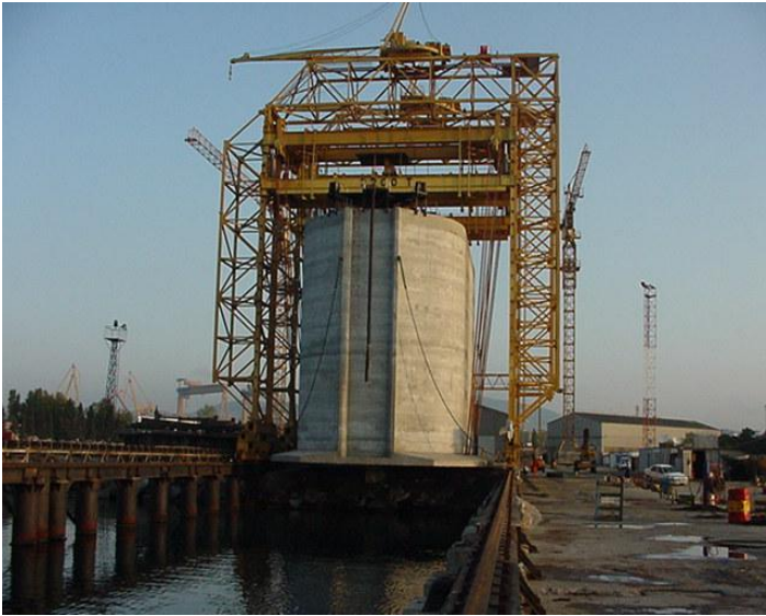
Figure 74: Handling of the Caisson
