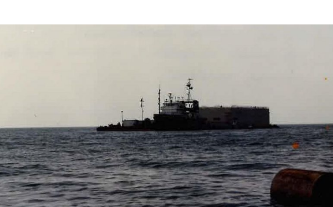
Figure 49: Towage of M. Ereğlisi LNG Terminal Caisson on the Ocean Going Submersible Barge of STFA (Koca Yusuf-II) by Ocean Going AHT of STFA(Yaşar Doğu-I). Courtesy of STFA Construction Co. (from CEng. Mr. Arif Yeşiltepe's Private Archive)
